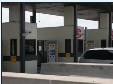
Fixed-mount LPR devices at tollbooth.
